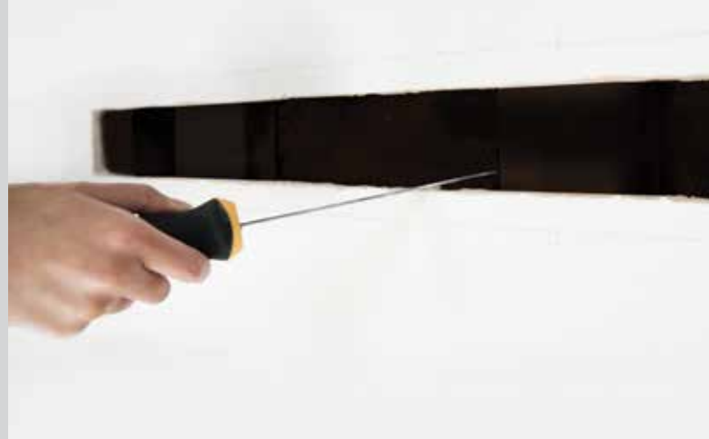
Step 2: Cut out 2 3/8" wide and 5/8" deep opening to the length of the channel run
