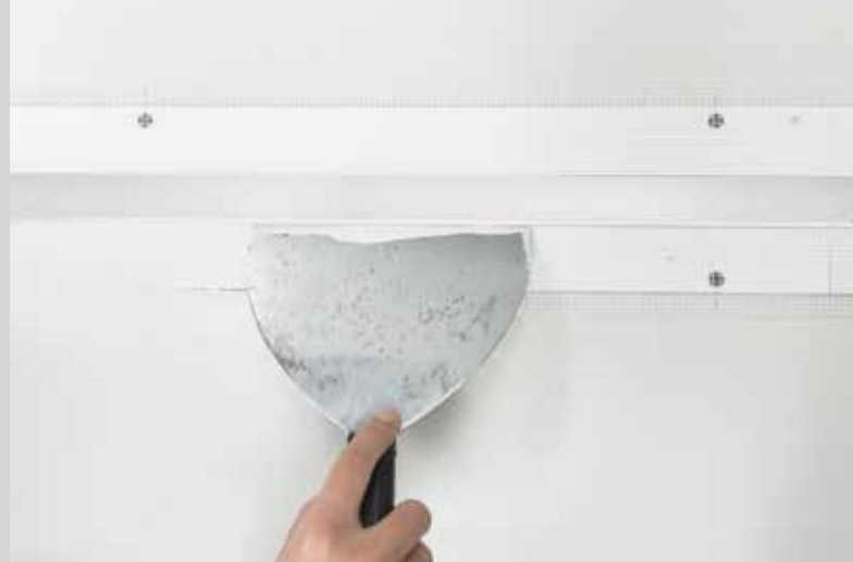
Step 4: Spackle, sand and paint around the soft strip channel
