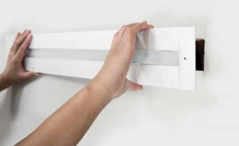
Step 3: Cut channel and mount channel to studs without removing the foam insert
