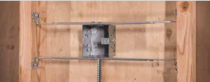
Step 3: Cut channel and mount channel to studs without removing the foam insert
